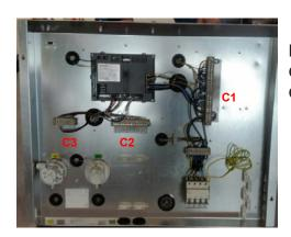
Each boiler has 3 terminal strips (C1..C3) and 7 cable guides.
