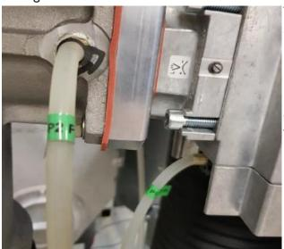
The tubing (PI & P2) and its fixation is part of the security of the boiler. During the inspection and maintenance also all the tubing and its fixations must be checked. Check for leakage and correct fixation. In case of doubt replace tubing and or fixation. After reconnection of the tubing check for proper functioning of the boiler and also check the input and CO/CO2 figures.
